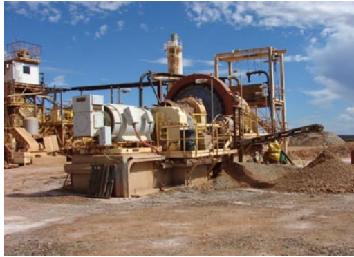
Lakewood gold processing facility
