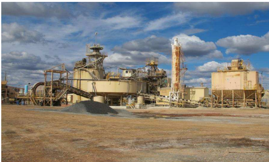
Exhibit 31: Lakewood processing facility
