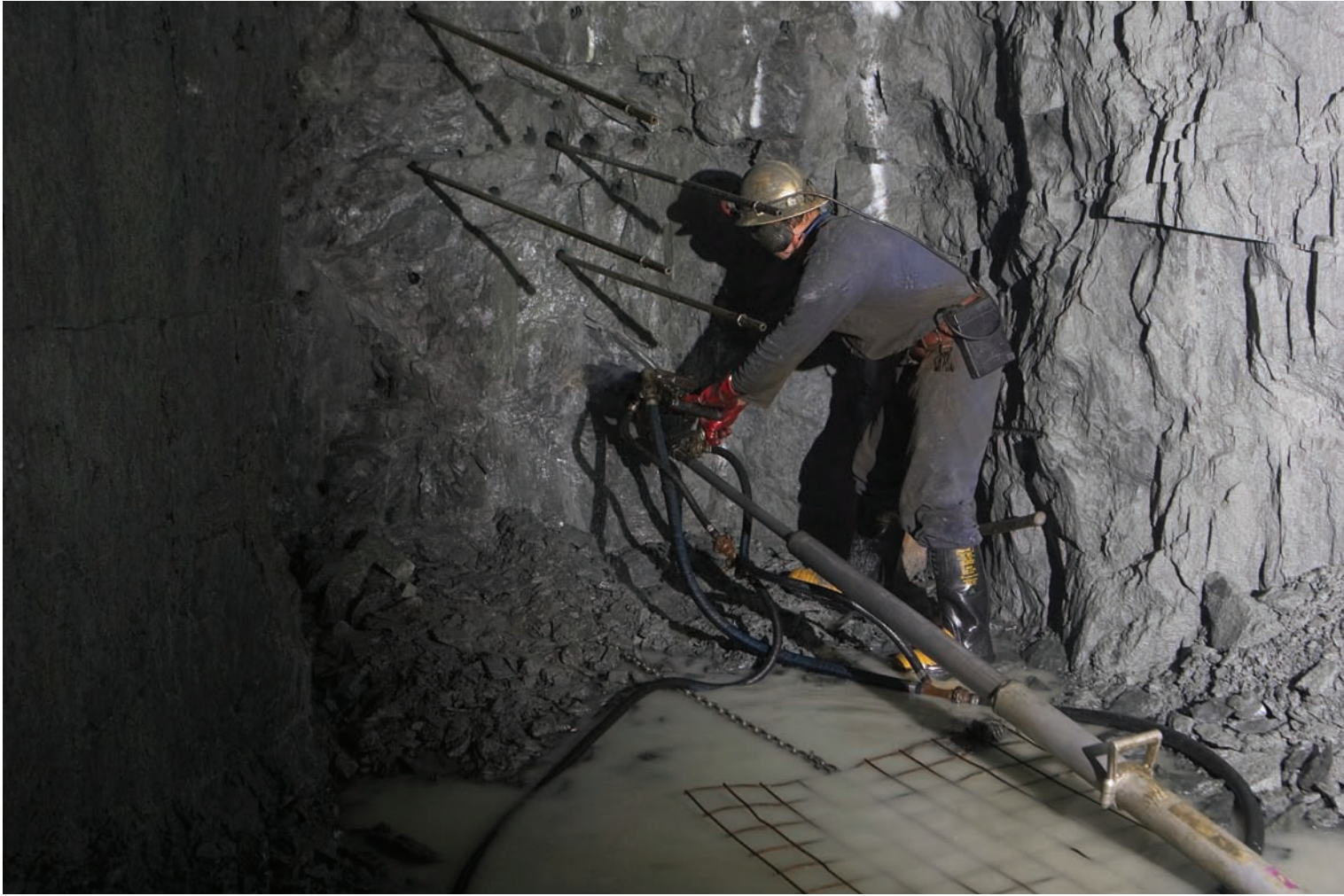
An Airleg miner drilling a face at Daisy Milano
