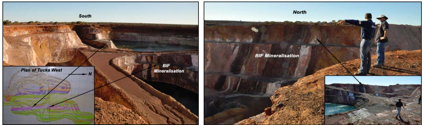
Figure 17. Views (South and North) of the BIF Mineralisation in the walls of the Tucka West Pit
